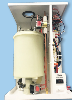
Front View, Face Removed
