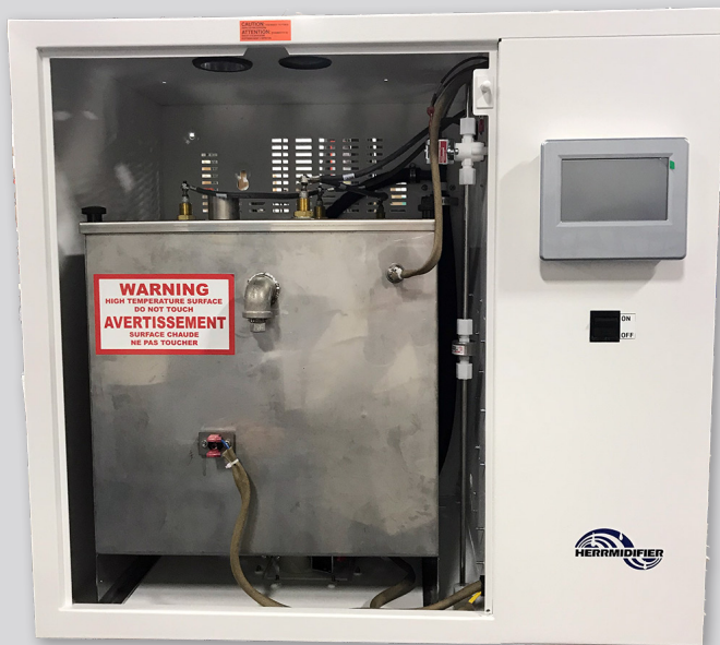
Front View, Face Removed
